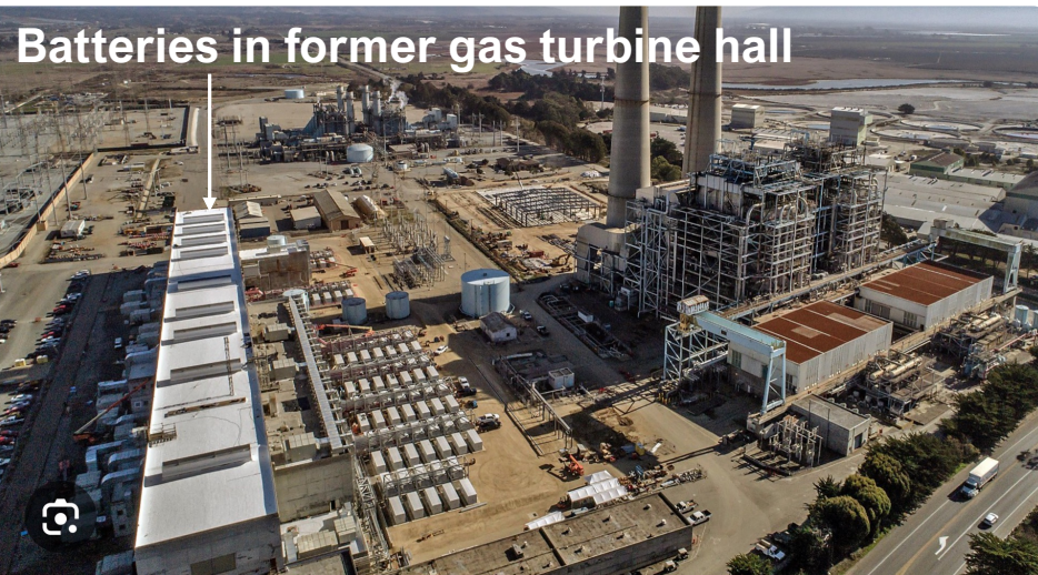
Moss Landing Battery Storage Plant in California (750 MW/3,000 MWh) Former fossil-fired plant converted to battery storage
